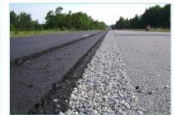
FiberMat® visible at center joint was exposed to 4th of July holiday weekend traffic with no reported issues
