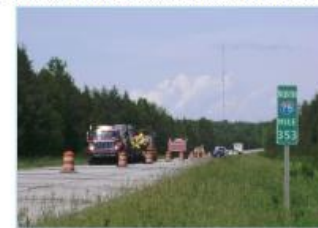
Strawser Construction placing FiberMat® on I-75 in Michigan's Ionia region
